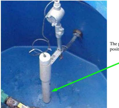
The photo at left shows a properly positioned sump sensor.
