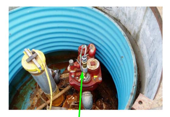
These two photos show different types of electronic LLDs mounted on top of STPs.
