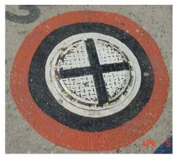
The photo at left shows a properly color-coded regular unleaded (containing a fuel extender) fill port with coaxial vapor recovery. The photo at right shows a properly colorcoded mid-grade unleaded (containing a fuel extender) fill port with dual-point vapor recovery.
