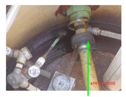
These two photos show test boots that have been properly pulled back after piping was tested.
