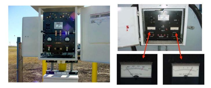
Above left – impressed current rectifier; above right – rectifier with both voltmeter & ammeter.
